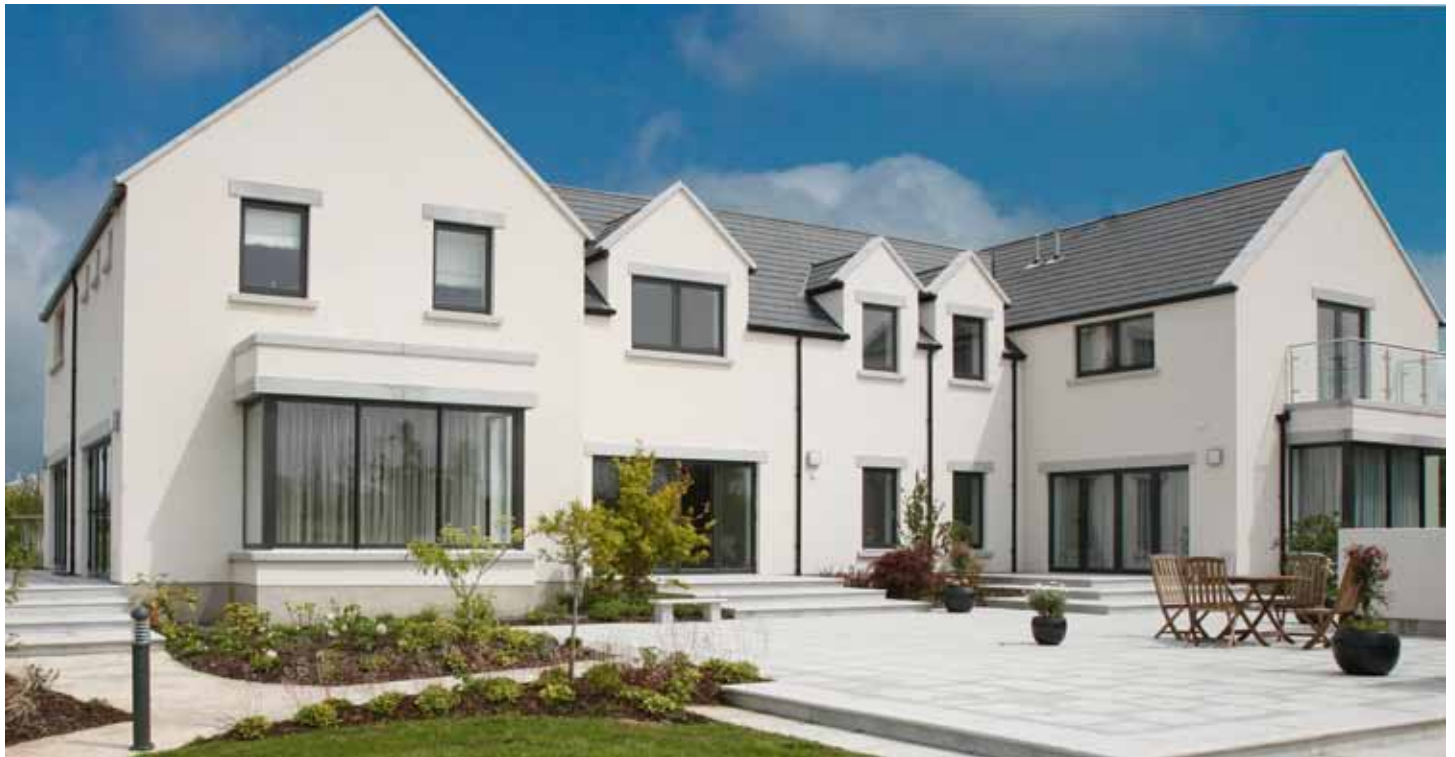
Top Left: House, Co. Antrim. Top Right: House, Cardiff. Bottom: House, Co. Down.
